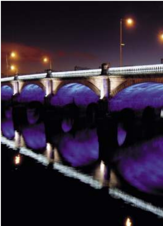
Glasgow Main Bridge, Scotland
