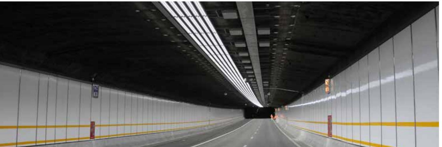
The superior colour rendering and higher perceived brightness makes it easier to distinguish objects and shapes. Drivers detect movement faster and from a greater distance with white light, giving them more time to react should the unexpected happen.
