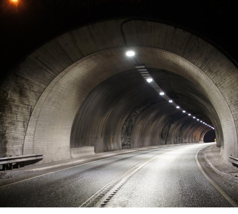
design, cable package and commissioning. It is a completely integrated lighting concept. The solution used in Ålesund consists of the TunneLogic control system and acidresistant FlowStar point source luminaires that provide good, consistent lighting throughout the tunnel.
