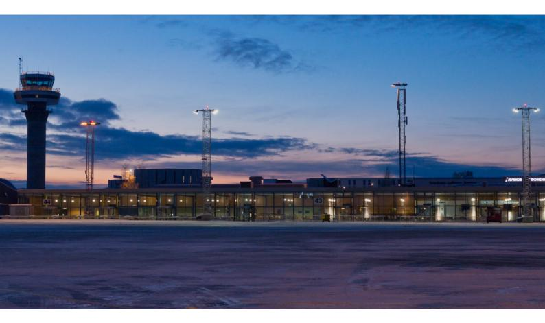
The installation delivered to Værnes consists of 18 OptiVision LED luminaires mounted on 6 high masts, 4 of which carry 2 luminaires each and use approx. 1 kW per high mast. The previous conventional installation at the airport used 4 kW per high mast, so a significant energy saving of  $\in$  12,944.84 per year is achieved versus the old installation.
