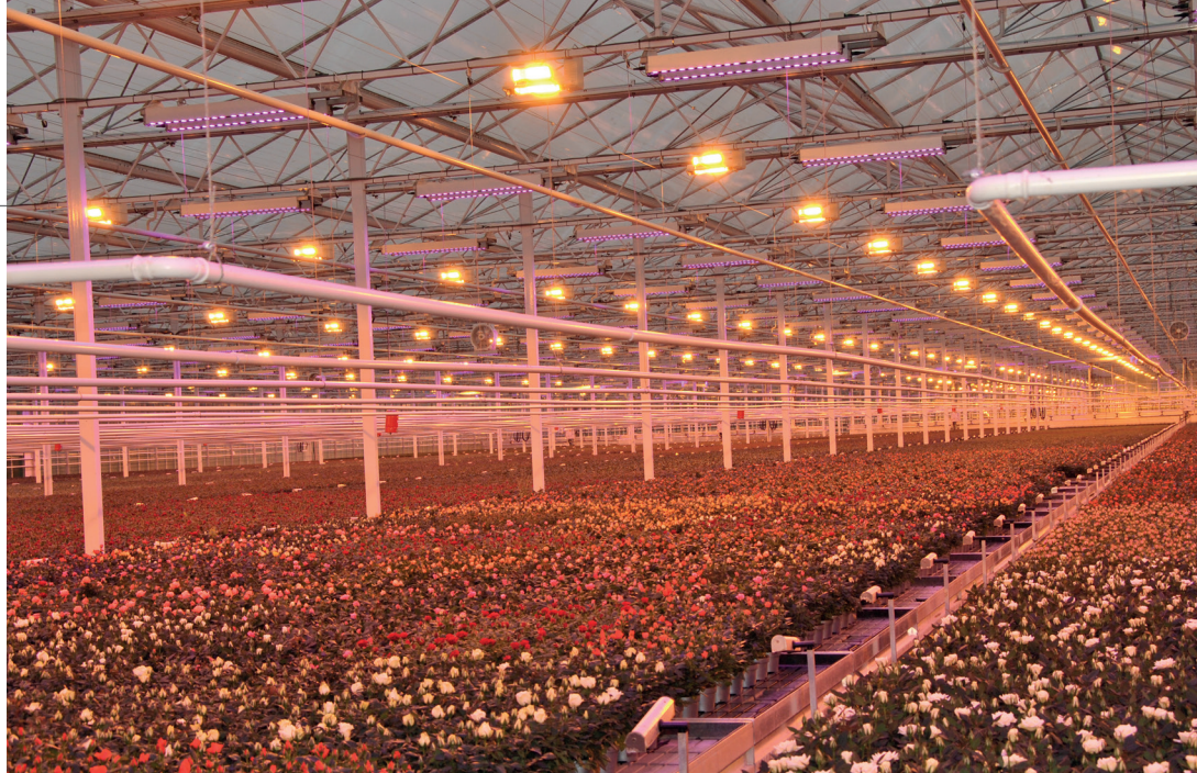
Last year, the first LED lights were installed in a newly constructed glasshouse block for finishing pot roses on Leo van der Harg's nursery.
