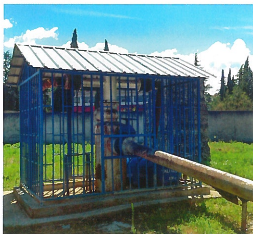
A geothermal heat source from the Soviet era heats the greenhouse.
