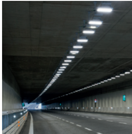
Tunnel interior lighting
