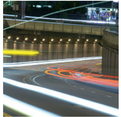
Tunnel underpass lighting
