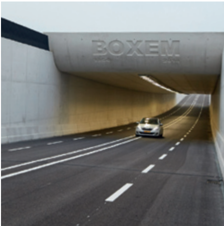
Tunnel entrance lighting
