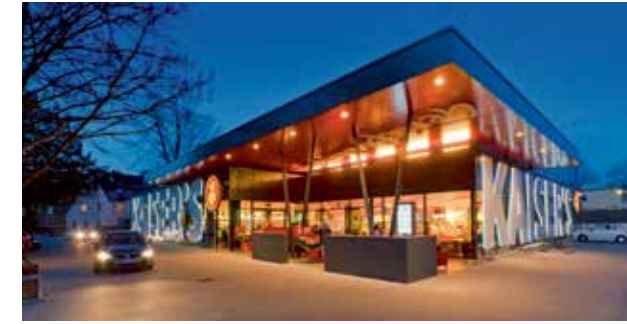
Outdoor parking and façade
