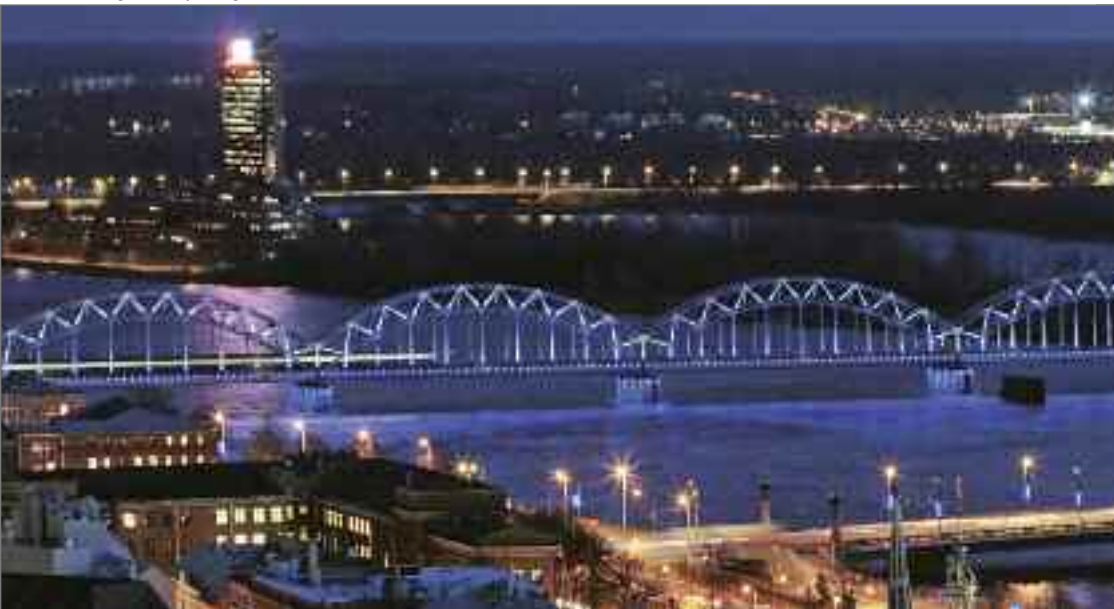
Latvia - Riga Railway Bridge
