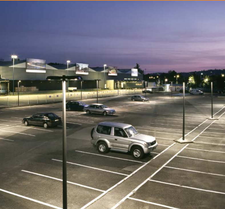
Flood light for carpark
