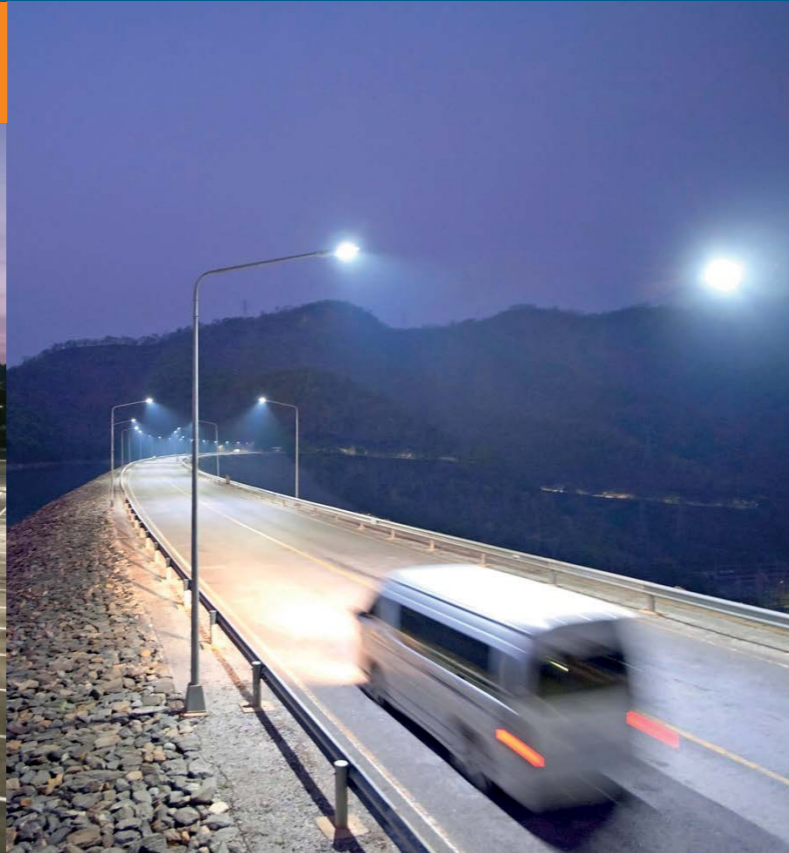
Streetlight for roads
