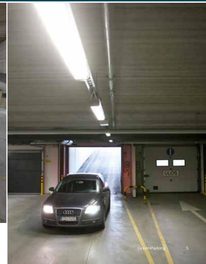
Both drivers and pedestrians benefit from uniform illumination as they move around the parking facility. Lights only come up to 100% when presence is detected. Otherwise, they dim to a fraction of full illumination.
