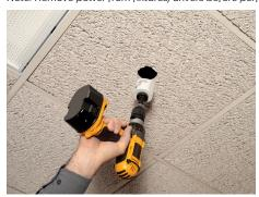
Step 1: Drill 2.5-inch hole in ceiling. It may be more practical to remove the ceiling tile and drill from the backside depending on material.
