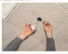
Step 2: Feed wires from sensor into ceiling hole. Wire length provided is 36-inches. Cable jacket provided is plenum-rated. Add additional wire length if necessary (18AWG solid wire recommended).
