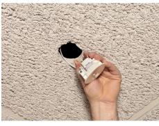
Step 3: Compress spring clips on sensor and insert into ceiling hole.
