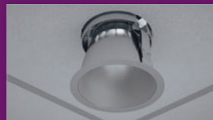
Reflector installs into ceiling.
