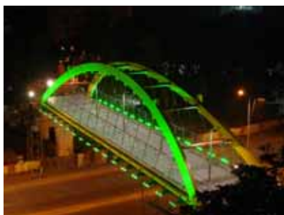
PSG College Bridge, India
