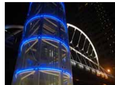
Banqiao East Hansheng Road Overbridge, Taiwan
