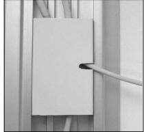
9.2 Press one side of the Cover into channel, routing cables behind Cover and through notches. Squeeze Cover and insert other side into channel.
