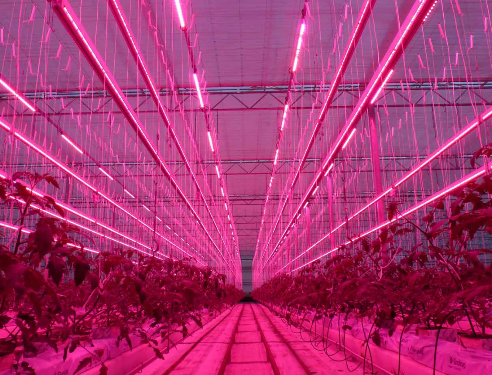
Double-row Philips GreenPower LED interlighting module and Philips GreenPower LED toplighting module
