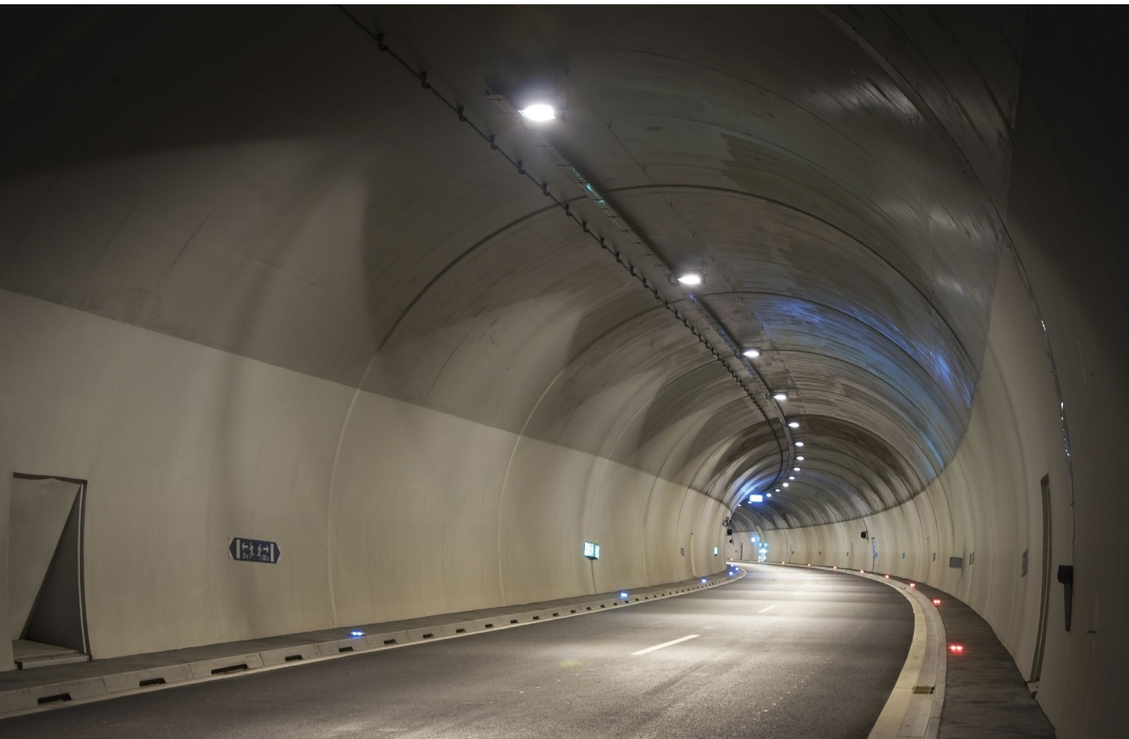
Emergency lighting at the side of the road in a traffic tunnel
