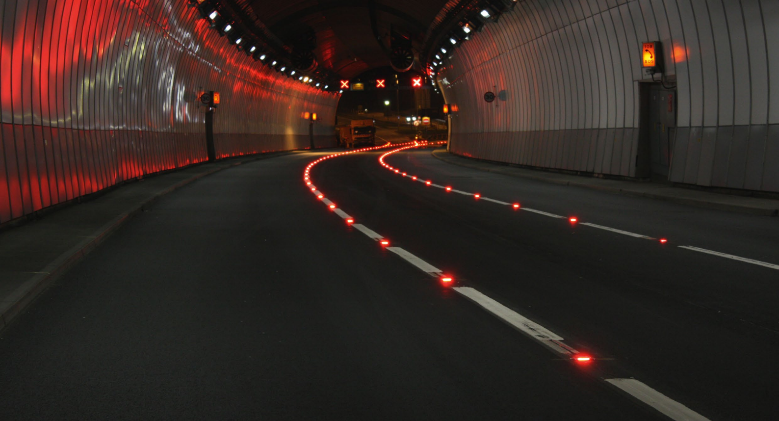
Saltash Tunnel, Cornwall, United Kingdom
