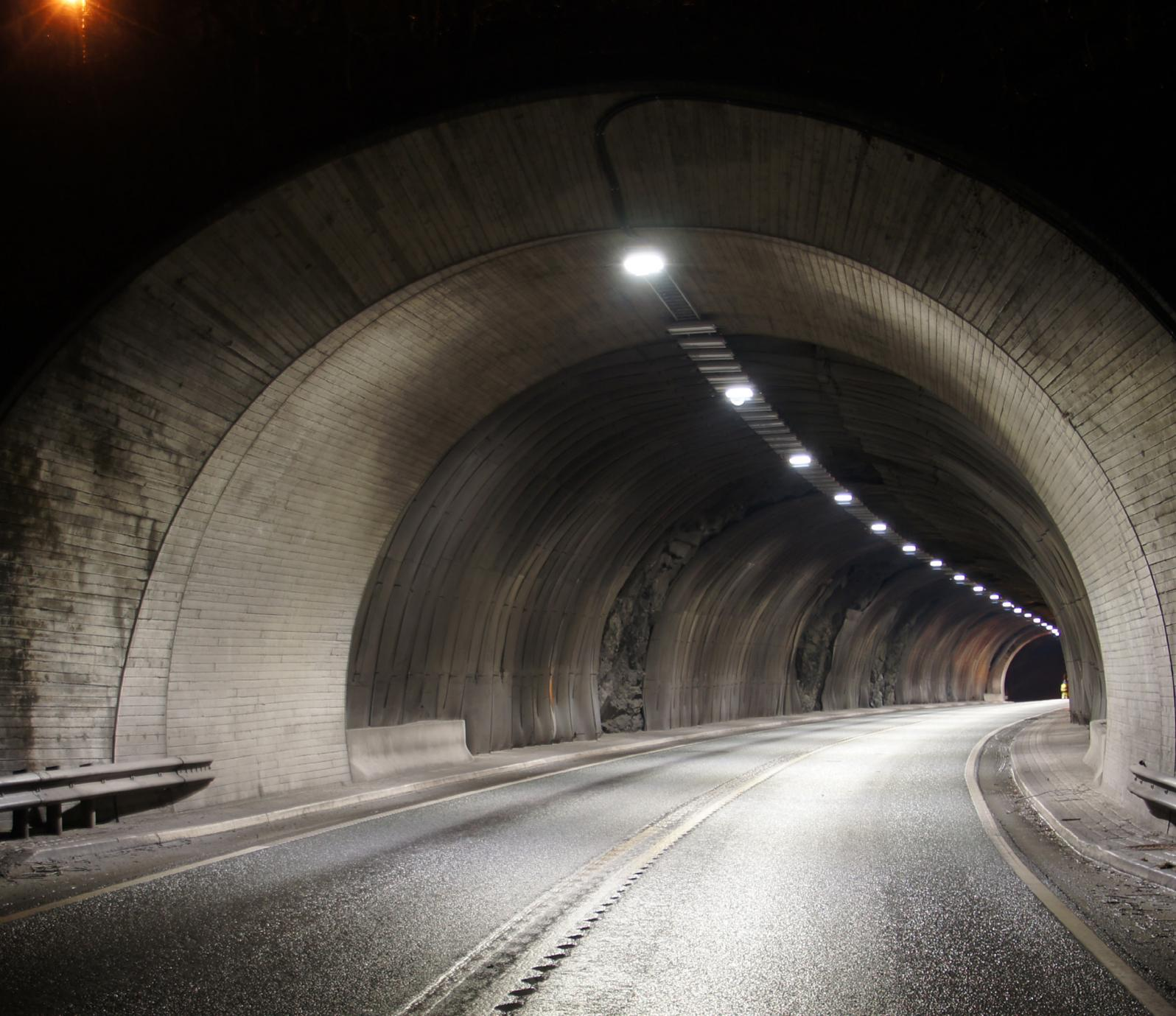
design, cable package and commissioning. It is a completely integrated lighting concept. The solution used in Ålesund consists of the TunneLogic control system and acid-resistant FlowStar point source luminaires that provide good, consistent lighting throughout the tunnel.
