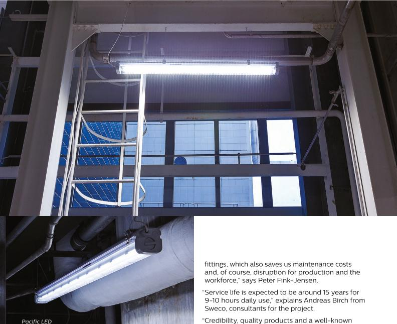
When no movement is detected after ten minutes, the light dims to 10%, and in designated areas switches off after a further ten minutes.
