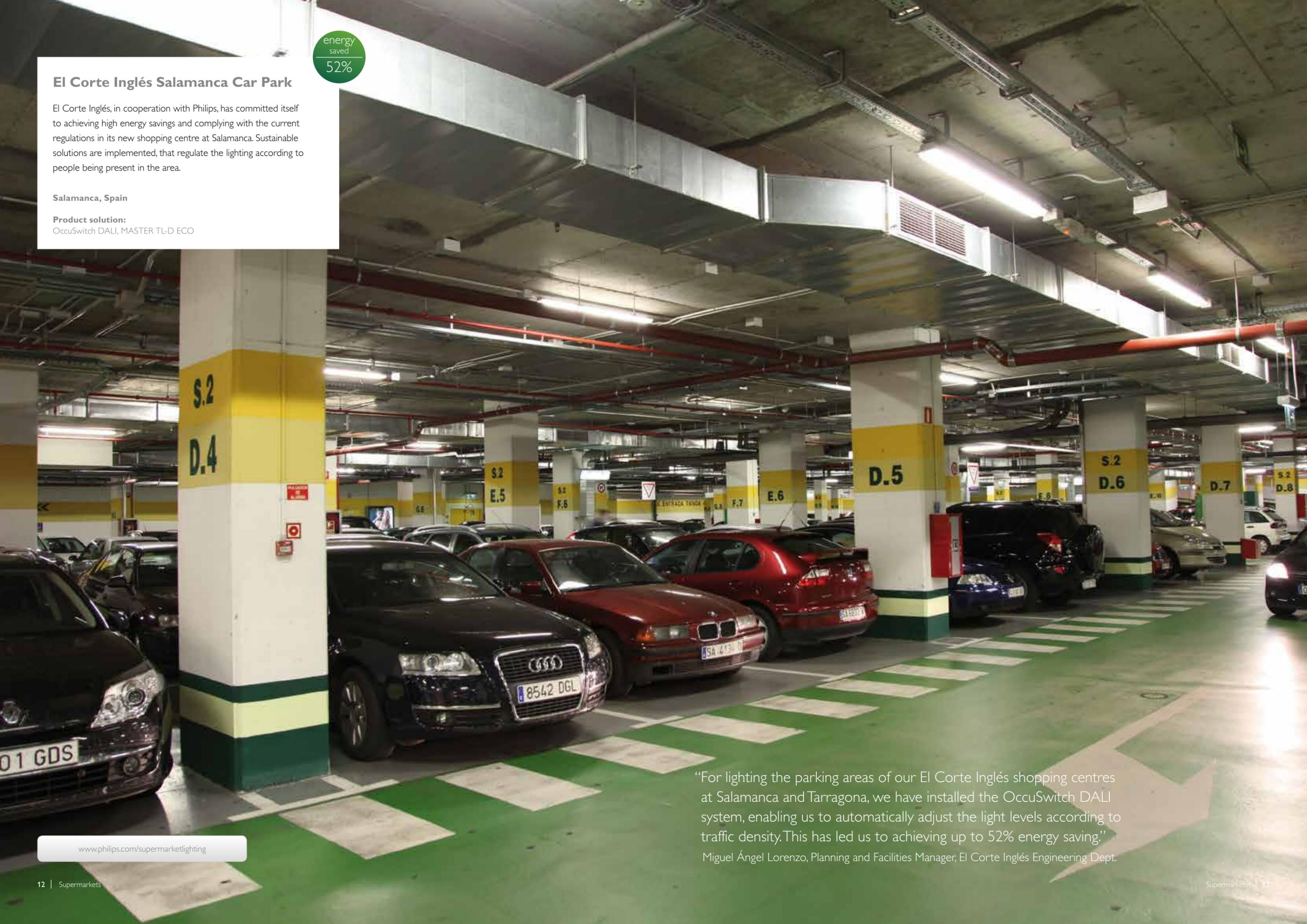
“For lighting the parking areas of our El Corte Inglés shopping centres at Salamanca and Tarragona, we have installed the OccuSwitch DALI system, enabling us to automatically adjust the light levels according to traffic density. This has led us to achieving up to 52% energy saving.”
