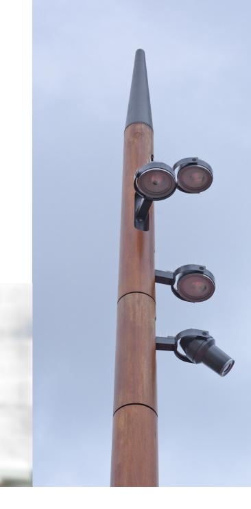
the structure as any movement of the column would impair the clarity of the CCTV pictures and for a while it seemed that timber would not be feasible. Then Philips calculated that we could use a steel column clad in timber to achieve the desired aesthetic effect." James Gordon continued.
