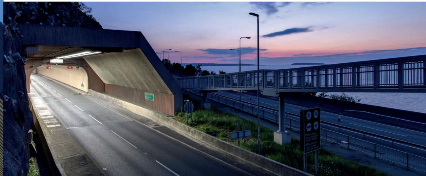
External photometers continually monitor these daylight levels and feed brightness data to the lighting controls, which instantaneously determine the correct corresponding lighting required within the tunnel.
