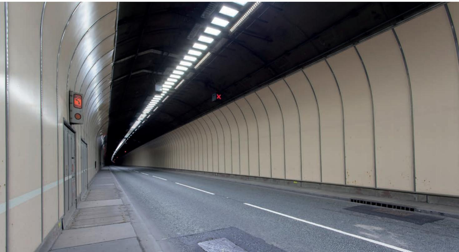
required new stainless steel primary fixing grid and cable trays. It also had to provide high lighting levels and uniformity in the threshold and transition zones and provide enhanced safety levels via dual redundant controls and adherence to rigorous fire safety requirements.
