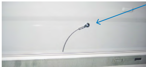
Picture H. Cable attached with self-drilling screw
